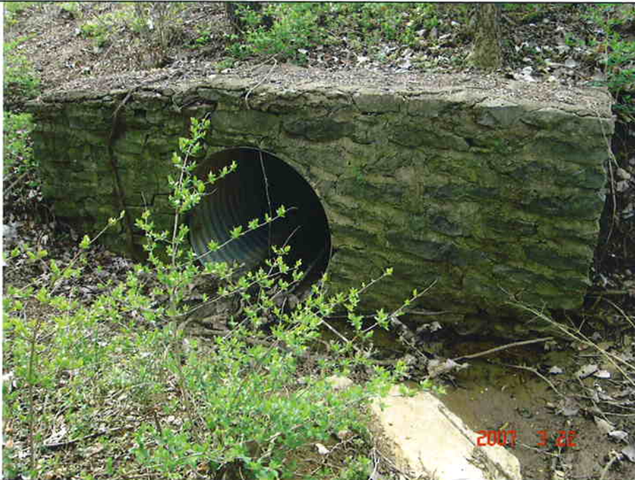
Photograph 12: Culvert that conveys STR-3, extends beneath Fairmeade Road.
